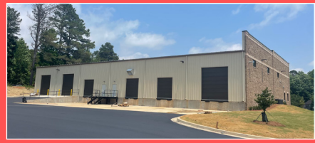
*Images show building at 6395 Cross Roads Road, which was delivered Q2 2023. 6395 Cross Roads Rd building is currently under construction, and will be of similar construction.
